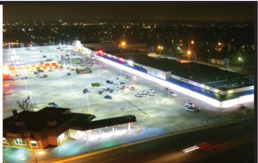
Phase II: Parking lot aglow with LEDs – project complete
