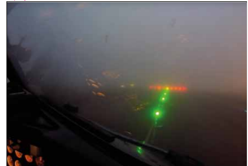
A full upgrade to the airfield lighting system will provide selectable routes for each individual aircraft between the runway and the gate, drastically raising the bar during low visibility operations.
