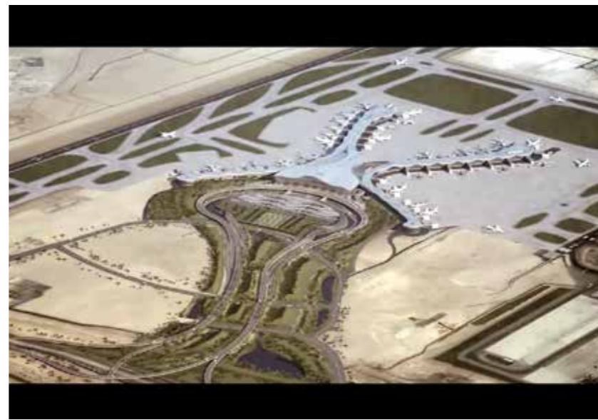
When completed, the MTB will be the third largest airport terminal building in the world, after Dubai and Beijing.
