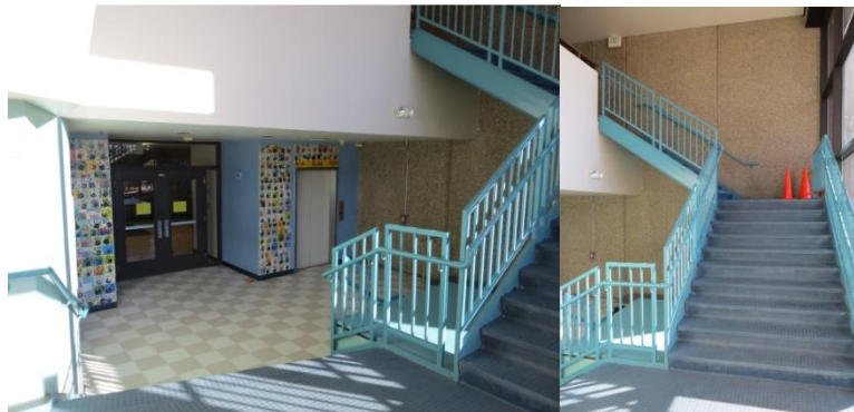
Main Entry Lobby- First Floor
