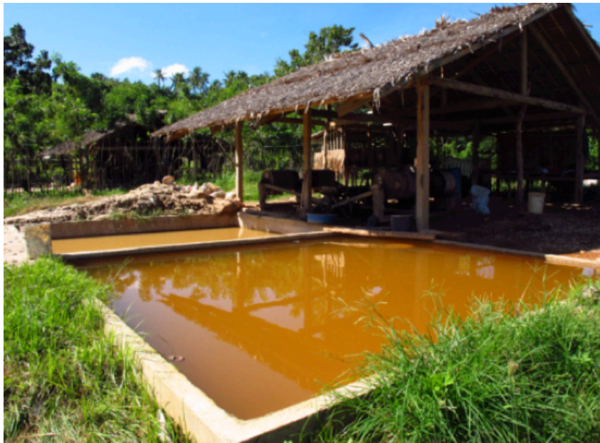
Figure 4. Tub. The tailings pond or Tub serves as a catch-basin for waste water from mining operations. Bigger dimensions for the tub prevent overflowing and ensure continued mining cycles.
