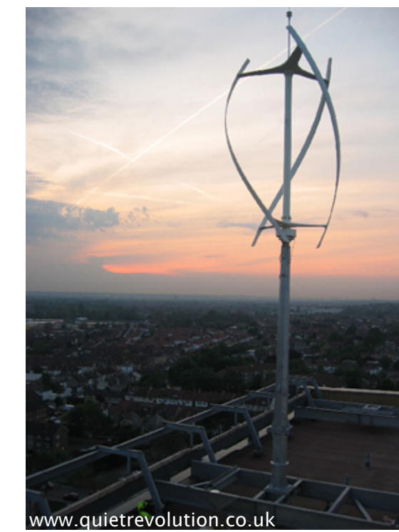
Board 3 3 The design of the Helical Wind Turbine allows power production with much lower wind speeds than the 3 blade wind turbine. Operating at lower wind speeds decreases noise and turbulence.
