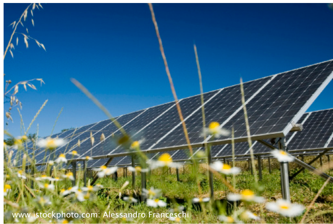
Board 3 1 The solar panels are sited on a south facing slope, which receives the most intense, direct sunlight creating the optimal conditions for power production.
