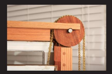
Four 275 link hand made chains are used to connect the reclaimed weights to the windows. The details where this occurs uses a multitude of seemingly impossible connections. Unique problem solving was used to make such a delicate looking portion so strong; able to take decades of abuse.
