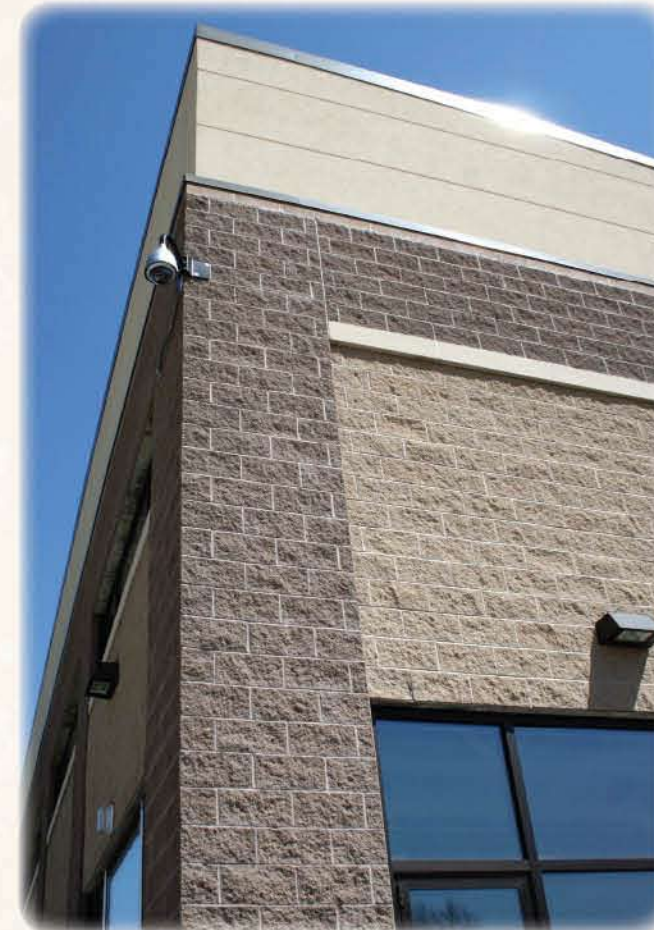
Above: Manheim Township High School, Lancaster, PA Split Face, Cocoa & Sandstone
