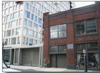
East Side of Building
