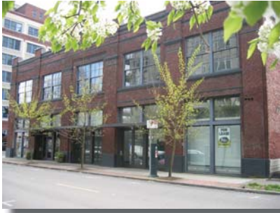
North Side of Building
