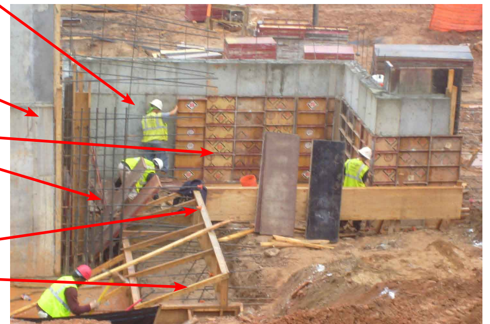
Observation of Form Liners being Removed
