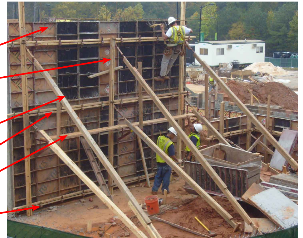
Observation of Form Liners and bracing
