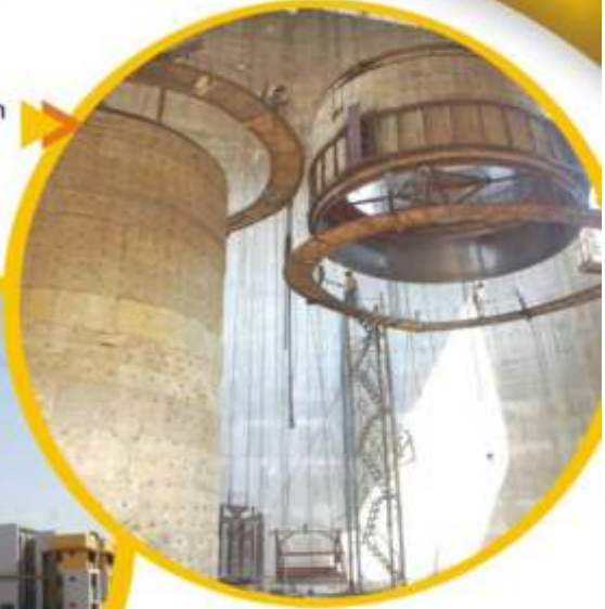
Flue can erection in progress
