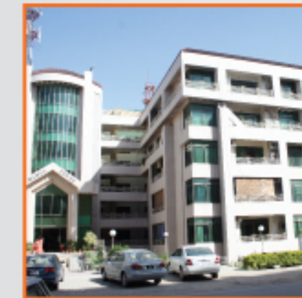
Hamza Tower Islamabad (Covered Area: 220000 Sft)
