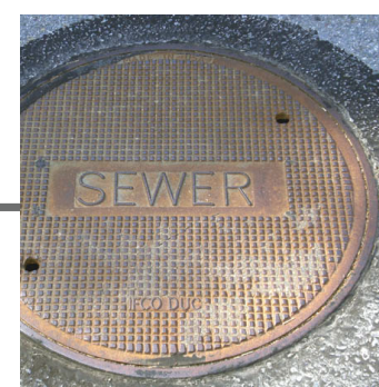
Water moves through 2,300 miles of sewer PIPE eventually hitting the dual 72" reinforced concrete pipes that head to the wwp
