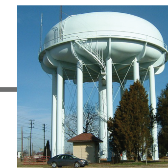
STORAGE tanks = 36 million gallons
