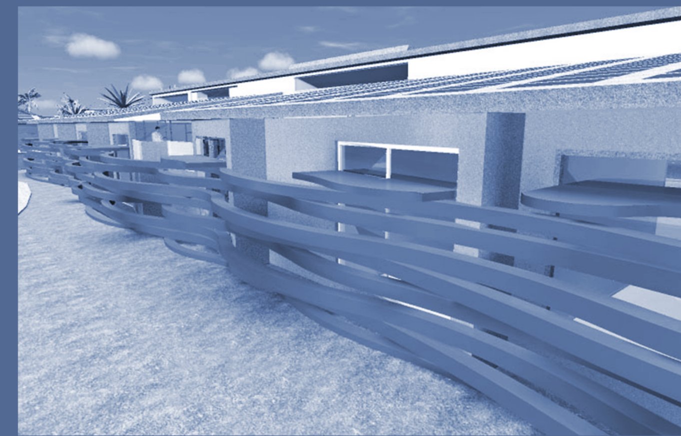
THE WAVE WALL LOUVER SYSTEM ACTS AS A WAY TO DIFFUSE SUNLIGHT AND SHADE THE LAB SPACES IN THE BUILDING, WHILE PROVIDING AN ELEMENT THAT LOOKS LIKE WATER TO THE BUILDING, CONNECTING THE DESIGN TO THE SURROUNDING ENVIRONMENT
