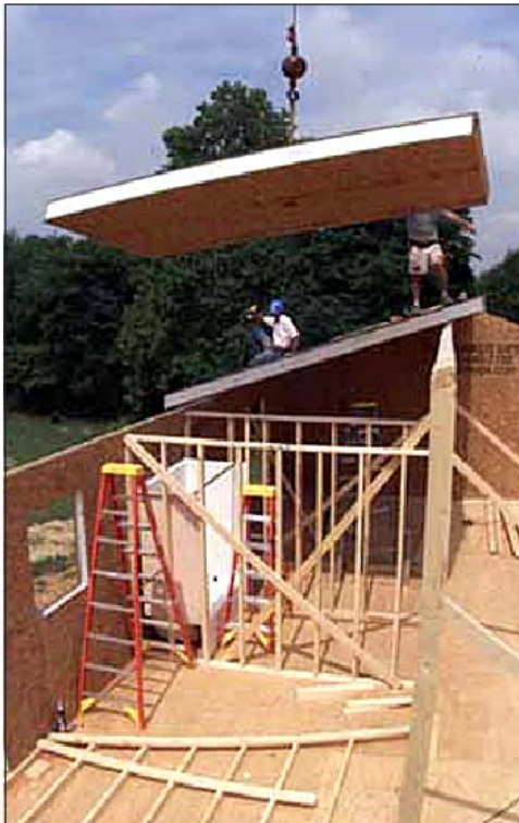
Image: SIPs construction at site
