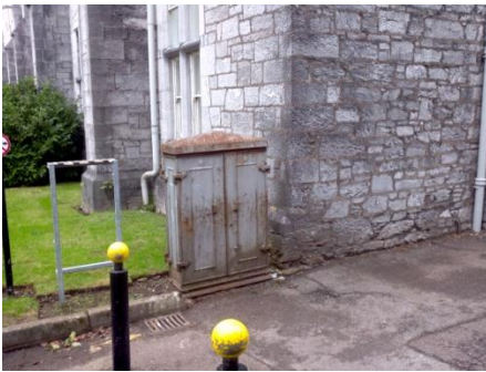
(Fig 2.1- External wall)
