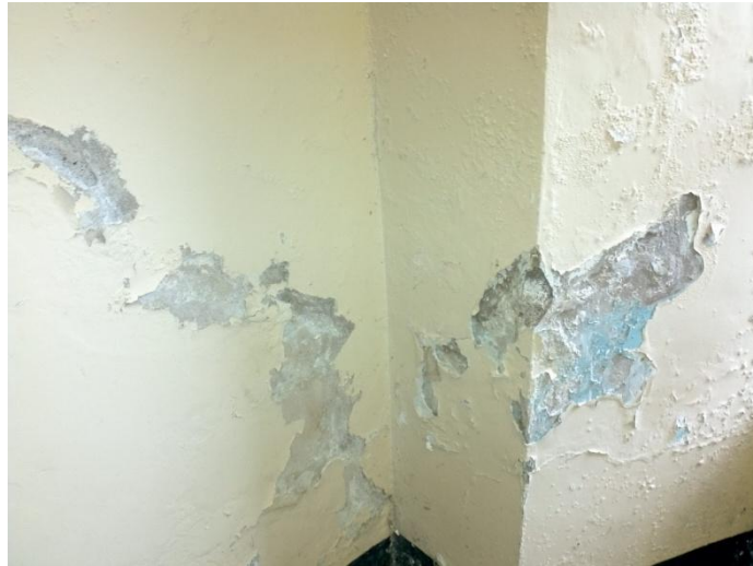
(Fig 3.3- Internal Plaster)
