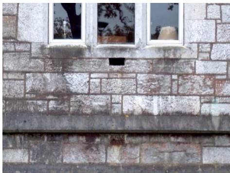
(Fig 2.3- External wall)
