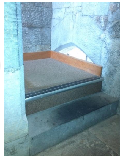
(Fig 2.12- Internal stairs)
