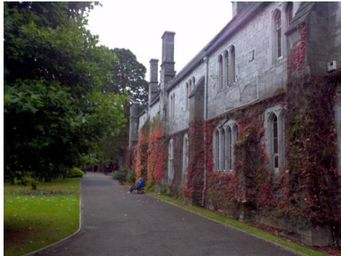
(Fig 2.5- External wall)
