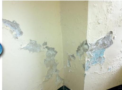
(Fig 2.10- Internal plaster)
