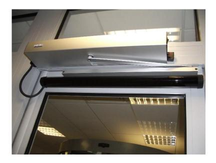
These door openers/closers can be controlled by either a sensor that will open it automatically or a push button that when pressed would open it automatically.
