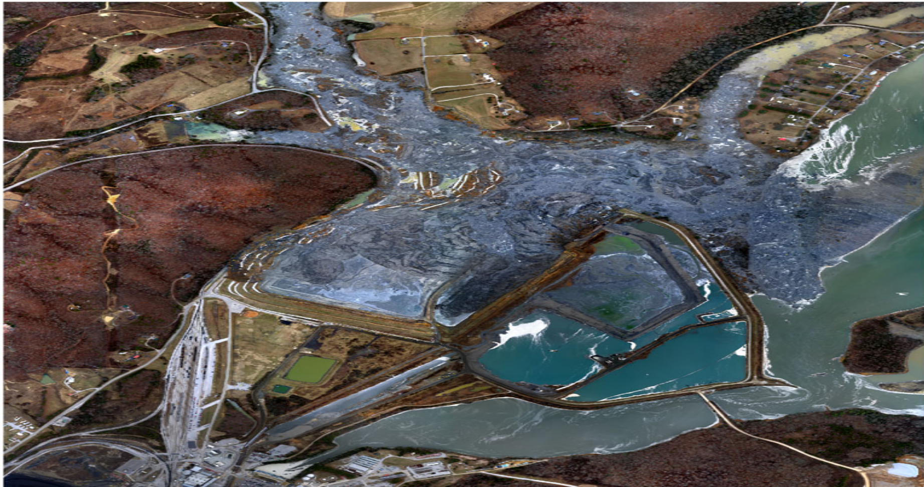
Aerial Image Of Kingston Ash Slide 12/23/08
