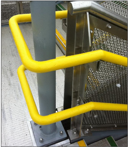
Handrail at Half Landing
