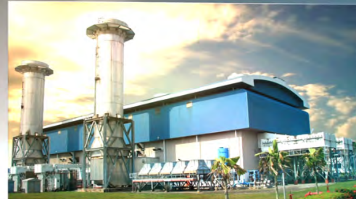
Bintulu Combined - Cycle Plant Total Capacity of 507MW
