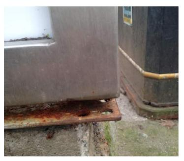
Most of the unsteadiness of the box is caused by missing bolts in the bottom sheet. Often this is because the metal has rusted though, but can be put down to lack of maintenence in other cases. Frames 100% locked down are impressively steady.
