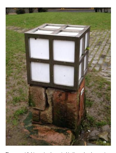
The current light was implemented in the redevelopment 25 years ago. Technical specifications are at the moment not apparent, and as a class, we haven't seen it being turned on. From what I can identify through observation, the box is constructed from sheet metal, with white plasic inserts.
