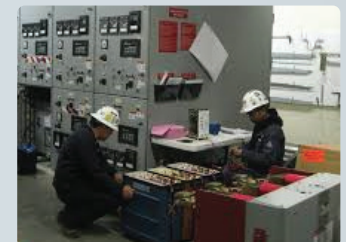
SWITCHGEAR REPAIR & MAINTENANCE
