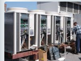
CHILLER REPAIR, MAINTENANCE & INSTALLATION
