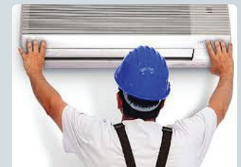
AIRCON/VRF REPAIR, MAINTENANCE & INSTALLATION
