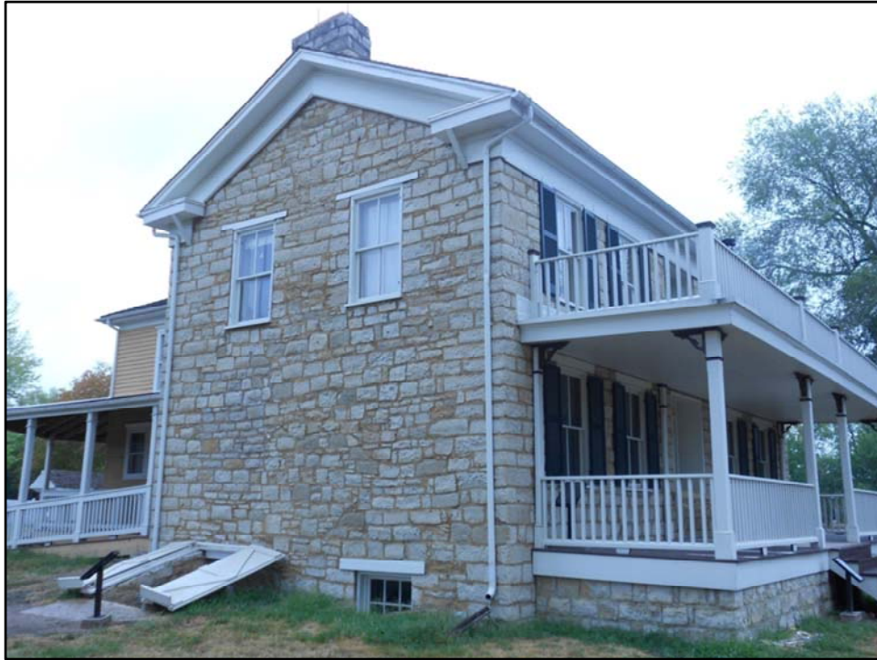
“The house was built of native limestone quarried on the property” (Lee, n.d.).
