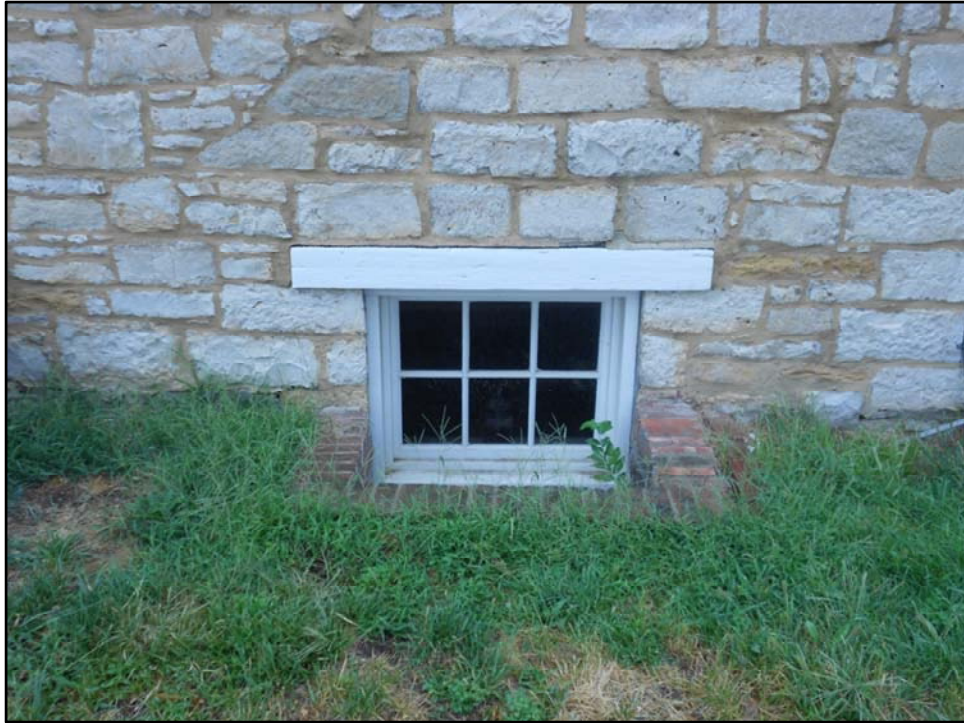
“A cellar window on the west side of the house.”
