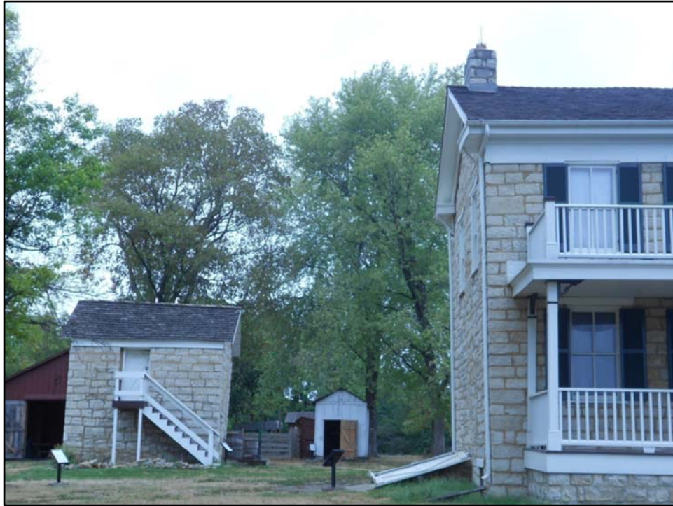
“Beside the house and to the rear stands the original ice house, also constructed of native limestone.”
