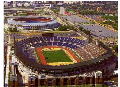
Top: The construction of the Olympic Stadium, now Turner Field Bottom: The finished Olympic Stadium
