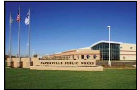
Naperville Public Works Facility Naperville, IL
