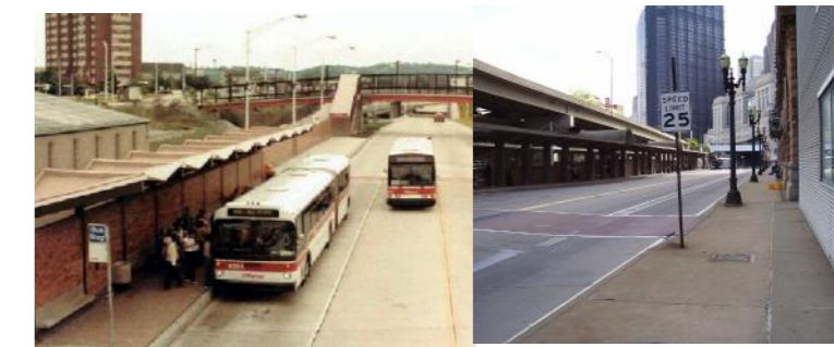
Martin Luther King Jr. East Busway, USA
