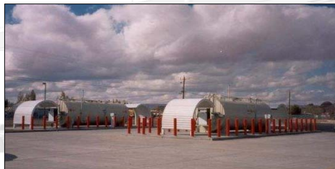
Kayenta Unified School District Refueling Facility
