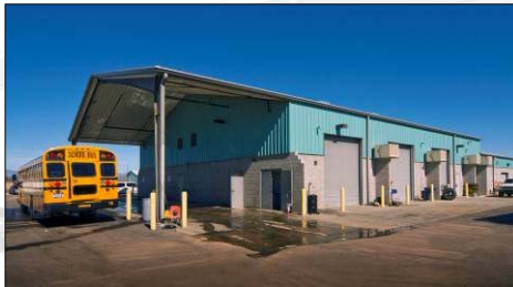
San Carlos Maintenance and Fueling Facility
