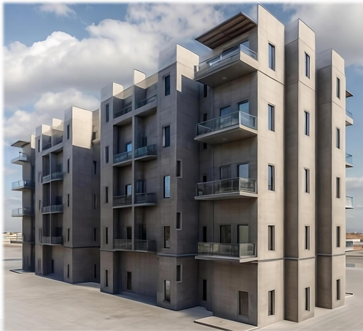
CORNER ELEVATION VIEW
