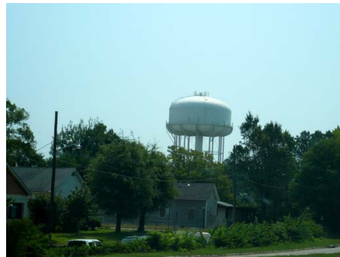
View of water tower
