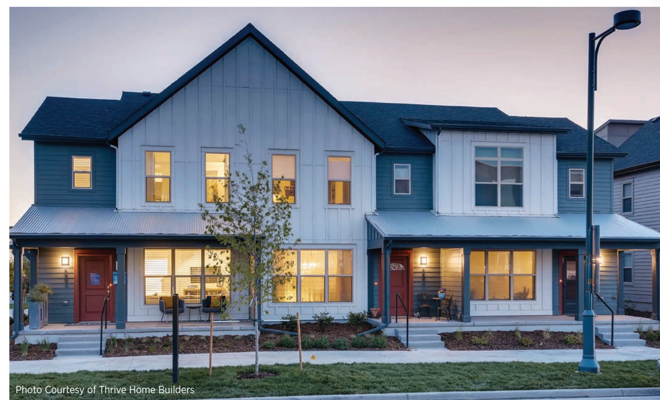
Production: This category recognizes builders who incorporate the DOE ZERH specs in consistent designs that can be cost effectively produced, like this production home in Denver built by Thrive Home Builders.
