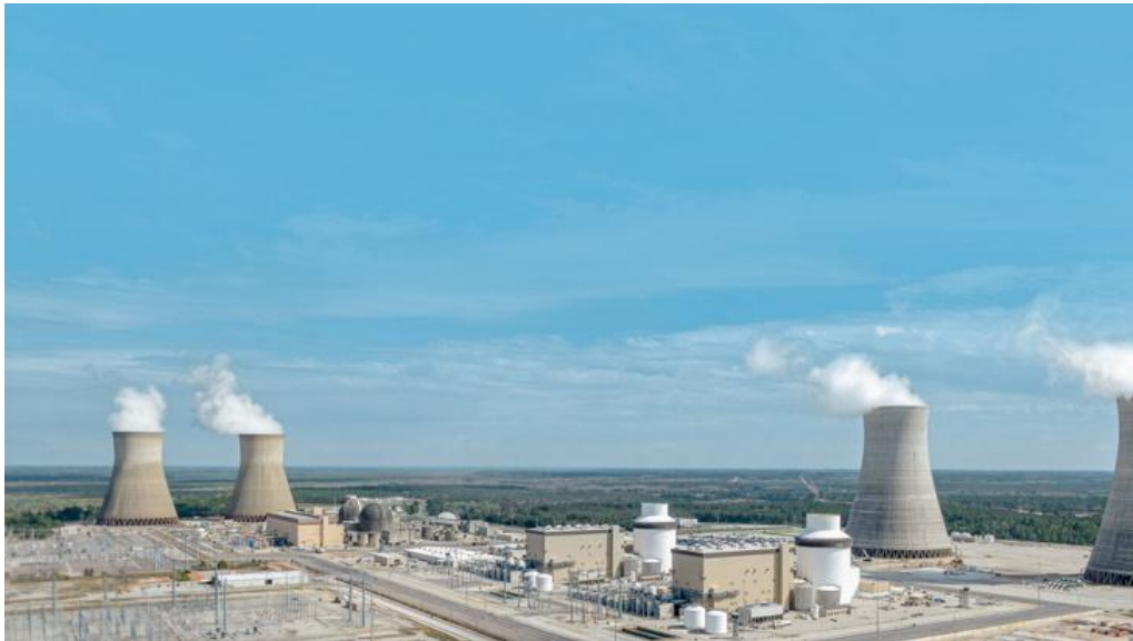
The four-unit Vogtle plant (Image: Georgia Power)
