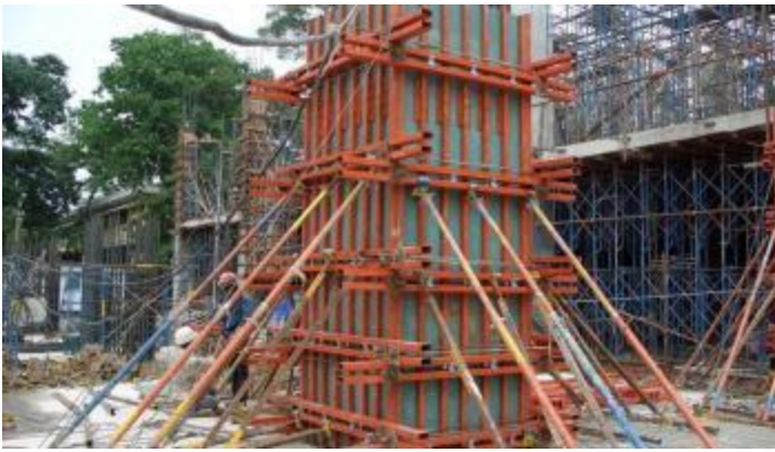
Concrete Formwork & Types of Formwork |Shuttering
