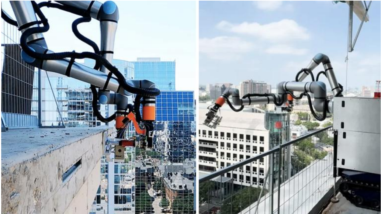
Robot completes critical tasks at 1,000 ft mid-air, 300% more efficient than manual labor
