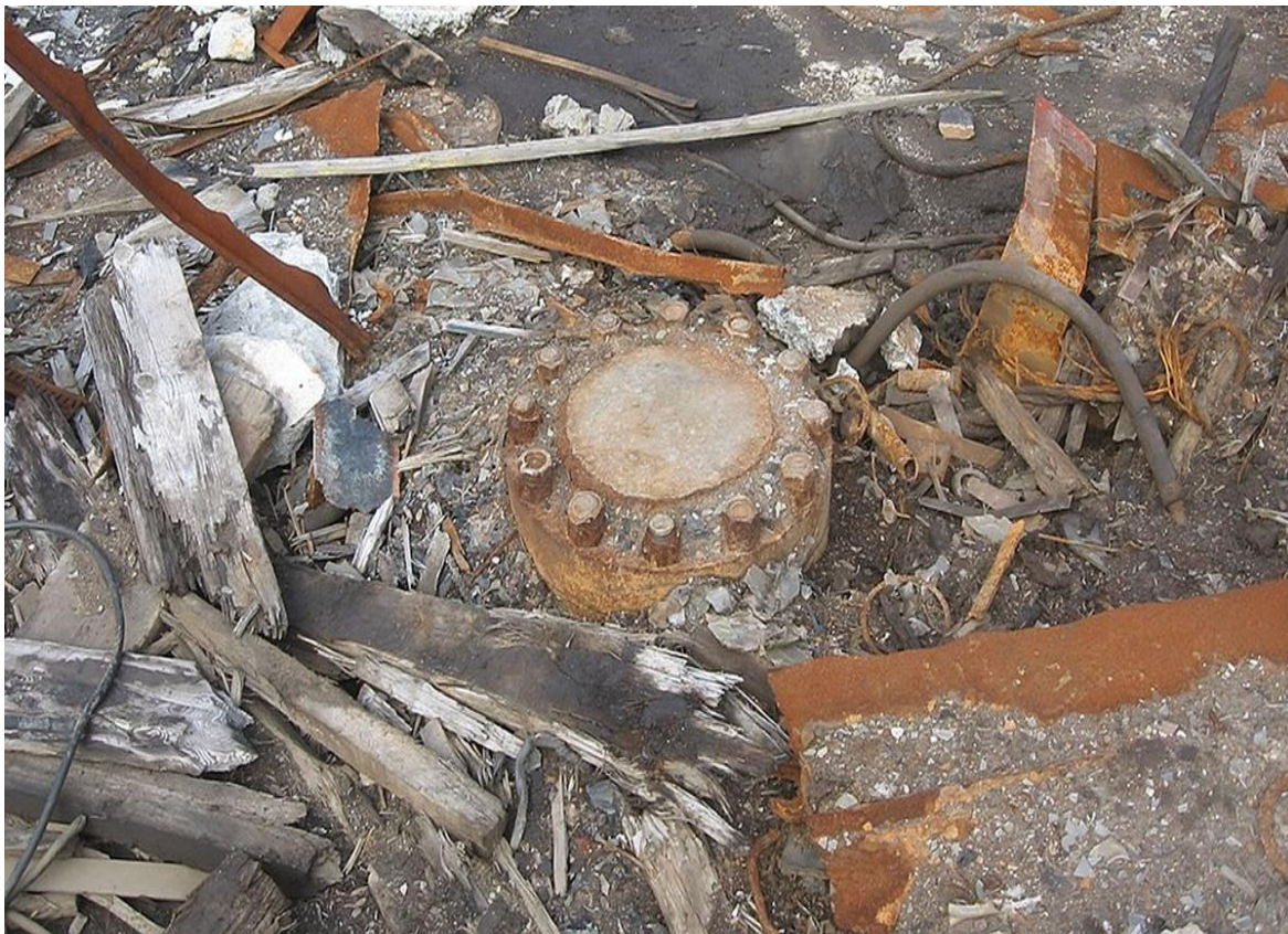
Image of the welded metal cap to the Kola borehole in Russia.
