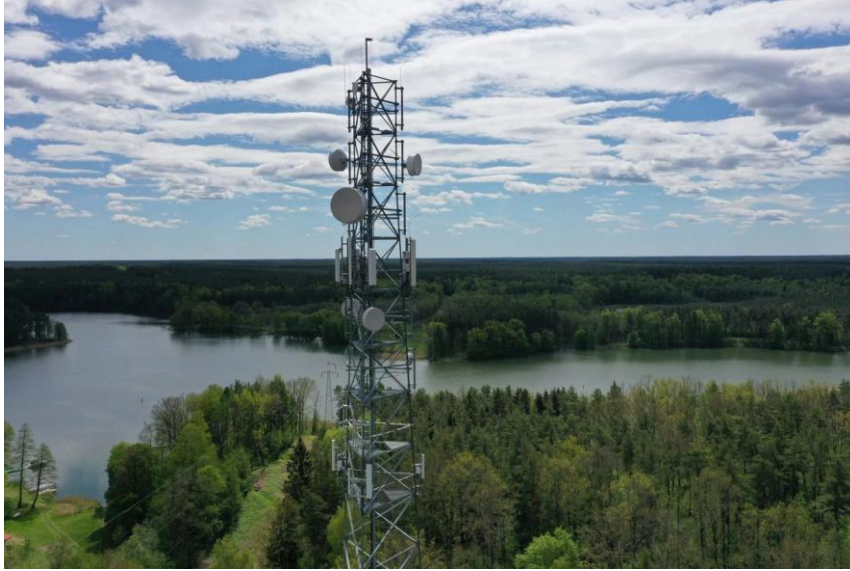
Base station (illustrative photo)
