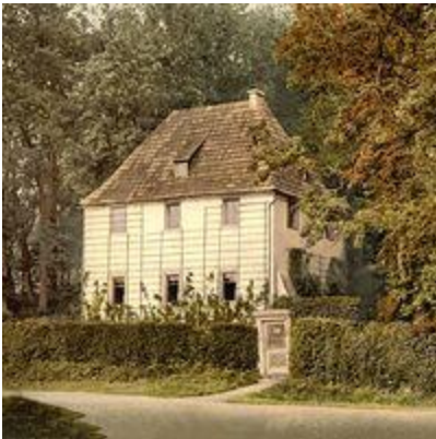
5 Historically Significant Houses in Germany
