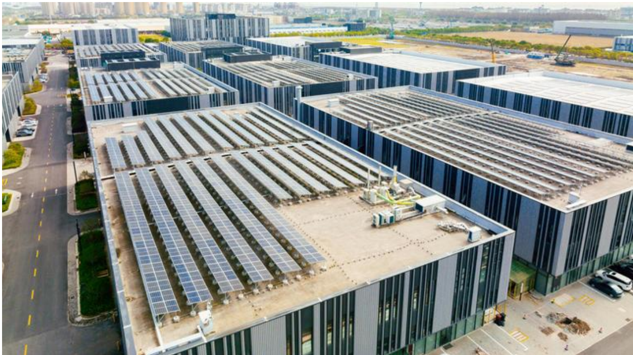
A view of several commercial roofs with solar panels© Asia-pacific Images Studio/Getty Images
