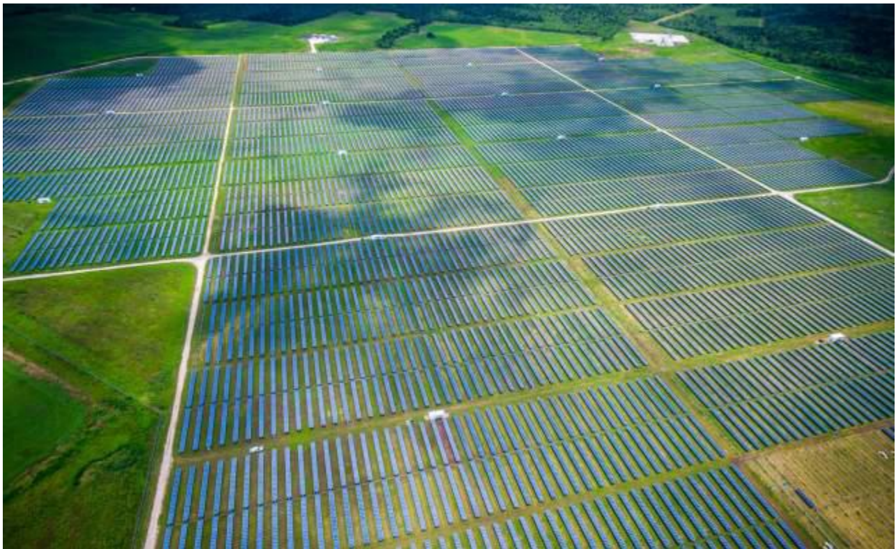
This solar-and-battery tag team means fewer worries about blackouts during heat waves and lower energy bills.
