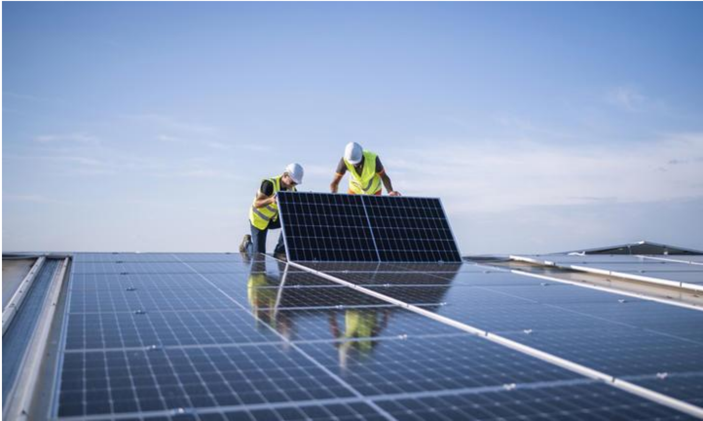
Solar panels getting installed© Artistgndphotography/Getty Images
