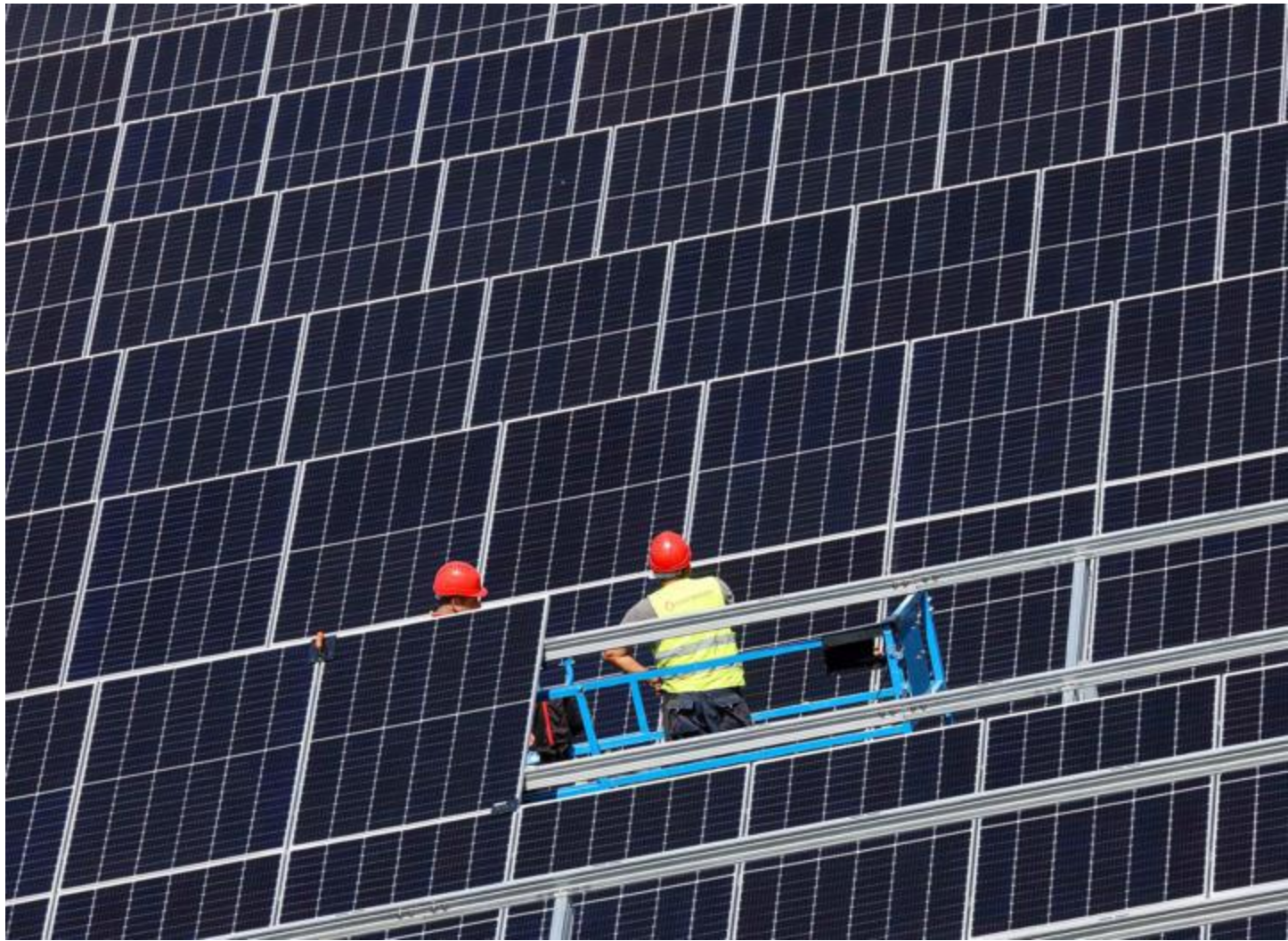
Workers install solar modules at the solar park in Langenenslingen, Germany, in August 2024. © Thomas Warnack / ZUMA
