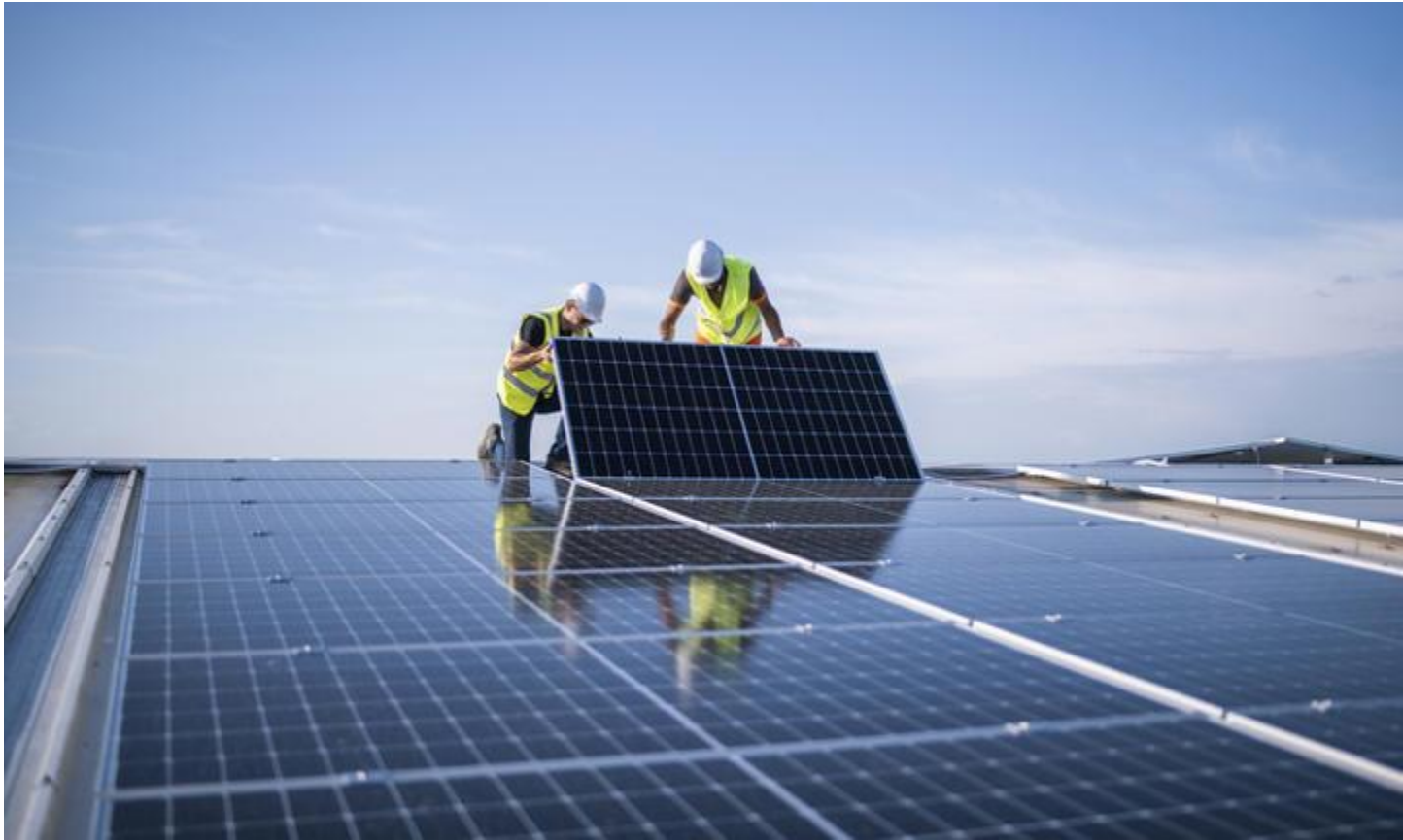
installing solar panels© Artistgndphotography/Getty Images
