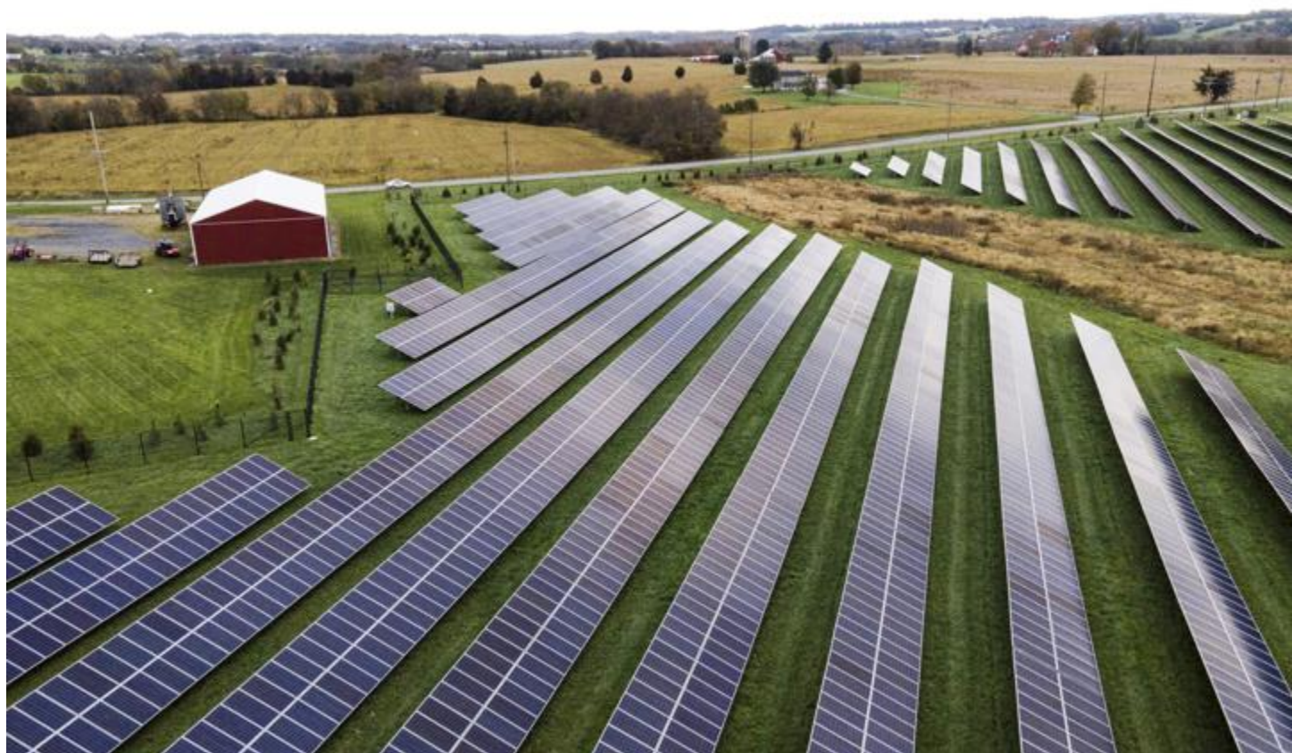
Solar panels that can generate electricity at night have been developed at Stanford© Jade Small
