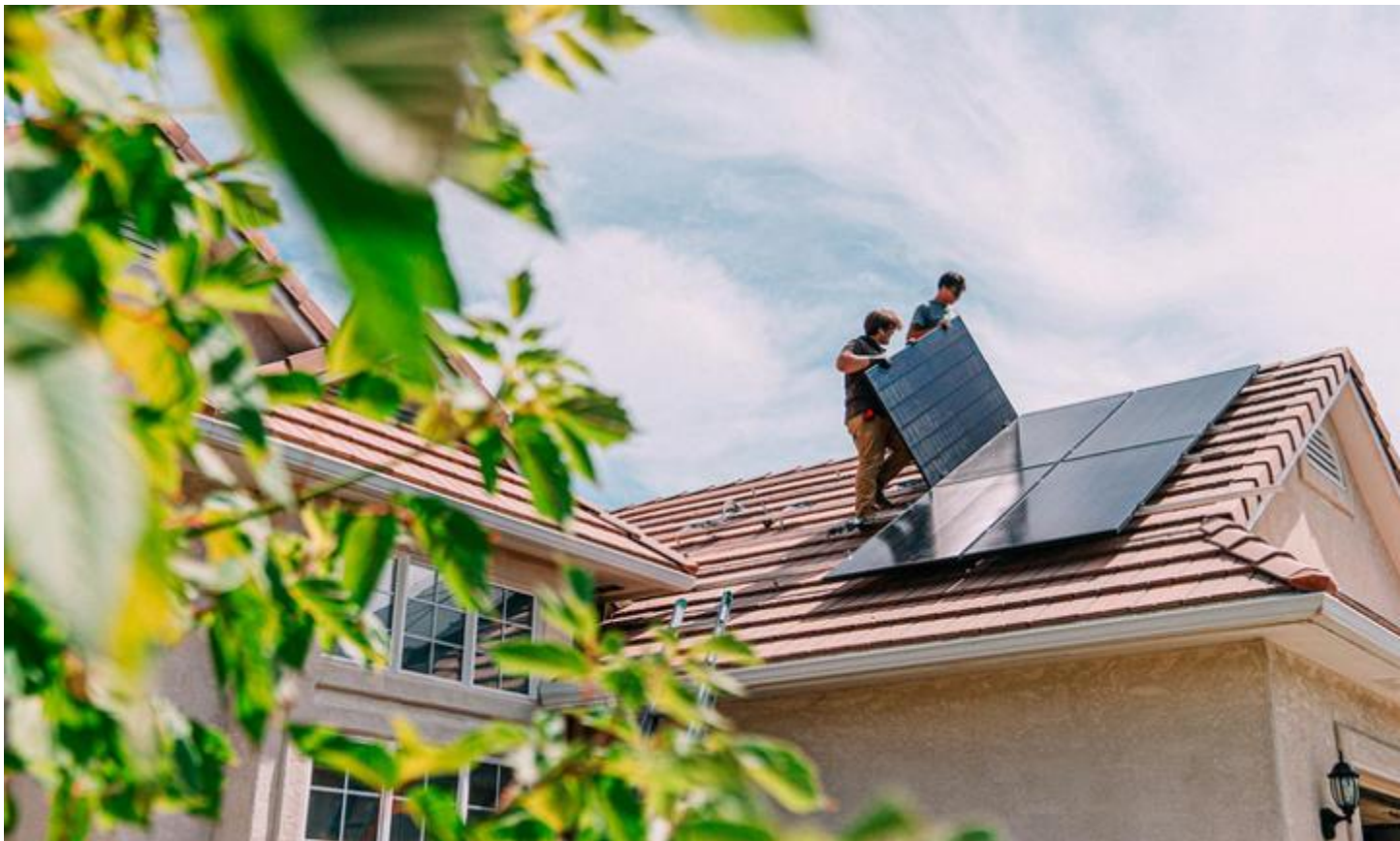
Men installing solar panels© Jeremy Poland/Getty Images
