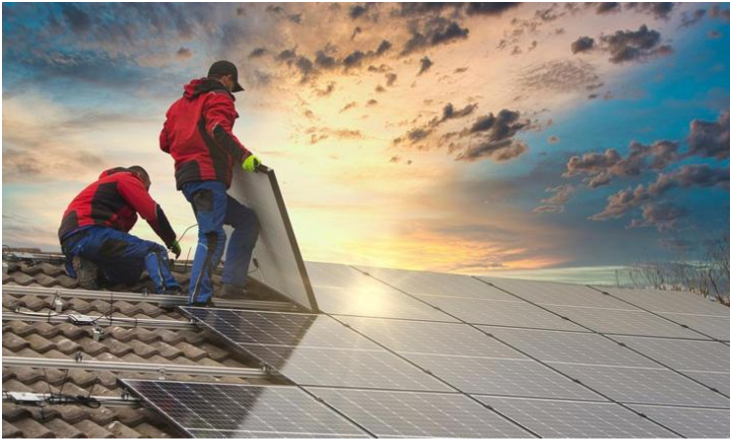
installing residential solar panels© moreimages/Shutterstock
