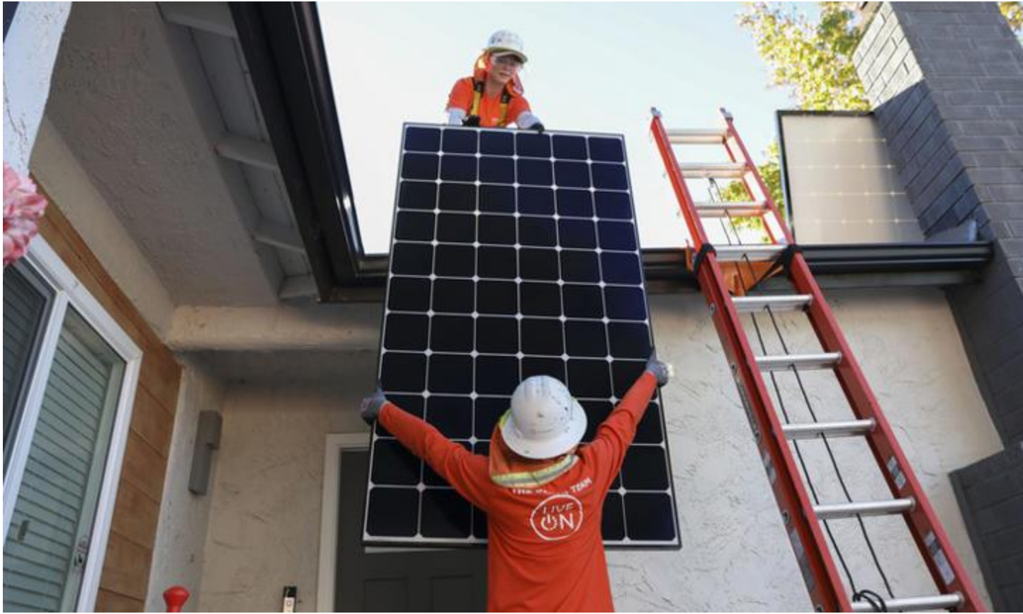
Workers installing solar panels on a home© Bloomberg/Getty Images
