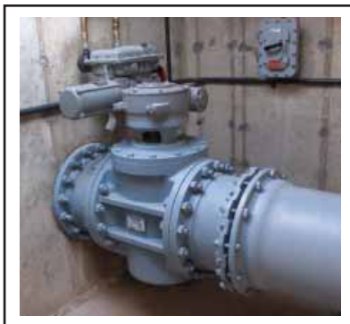
Cam-Centric® Plug Valve with motor actuator
