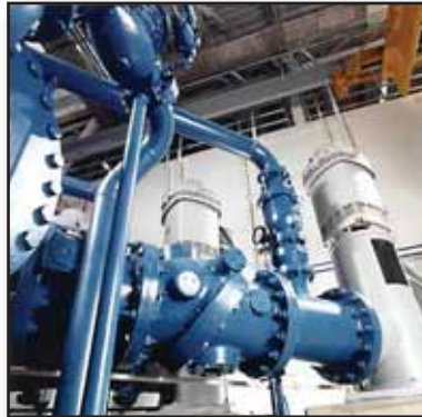
Tilted Disc® Check Valve with Well Service Air Valve on Vertical Turbine Pump.
