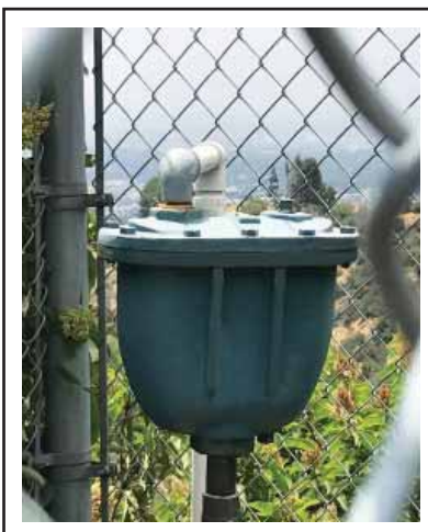
Single Body Combination Air Valve
