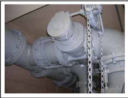
Cam-Centric® Plug Valve with worm gear actuator and chainwheel
