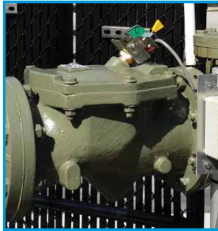
Swing-Flex® Check Valve with Limit Switch
