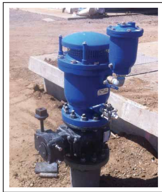
Dual Body Combination Air Valve
