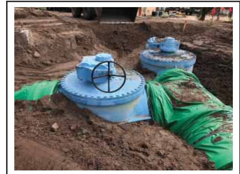
Cam-Centric® Plug Valve with worm gear actuator
