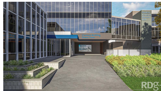
Courtyard view with new link
