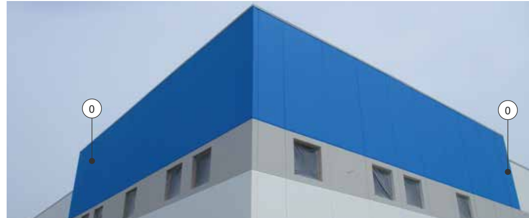
2 PHOTO EXISTING CONDITIONS
