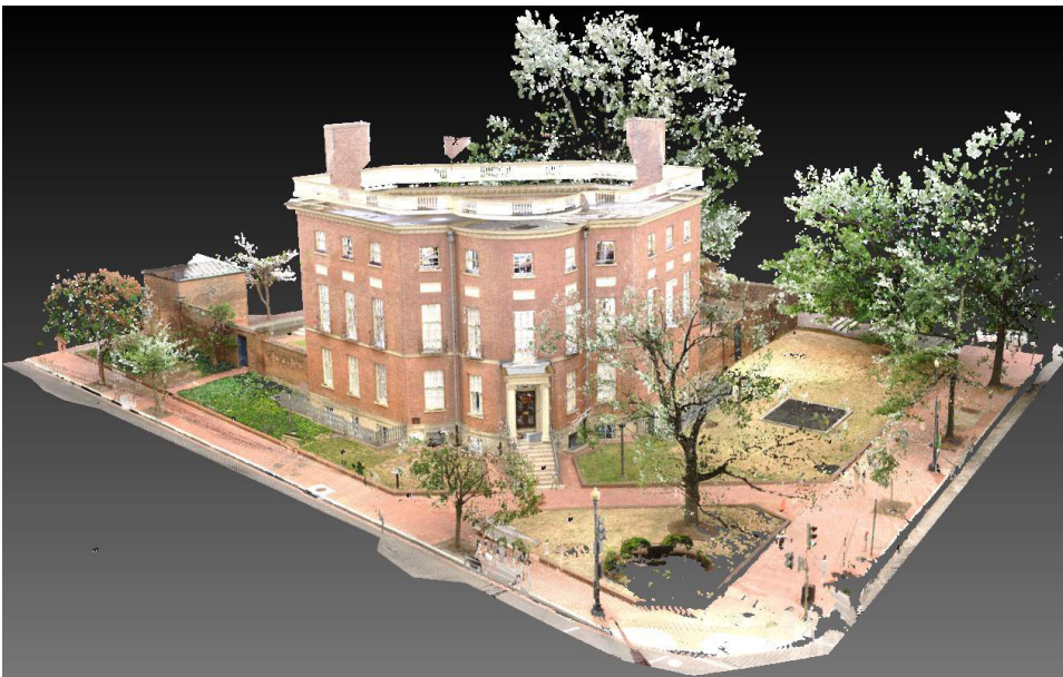
True Design Services captured the historic Octagon in Washington, D.C., using a FARO® laser scanner.
